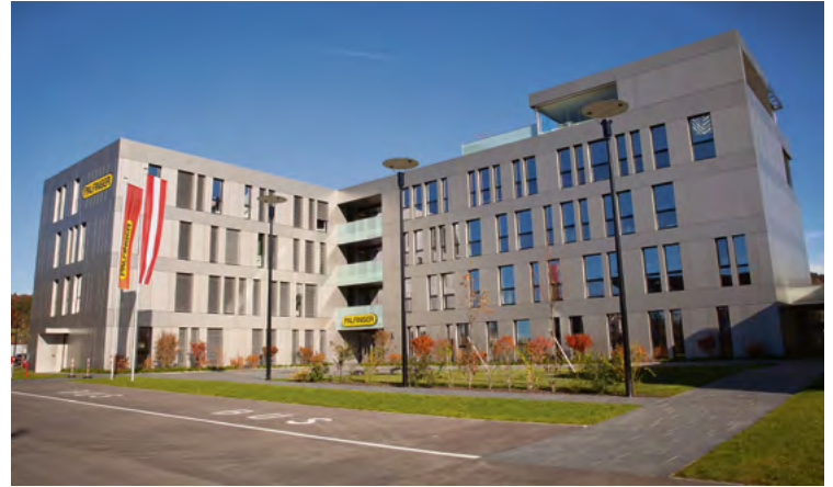
Das Palfinger-Headquarter in Salzburg-Bergheim.
